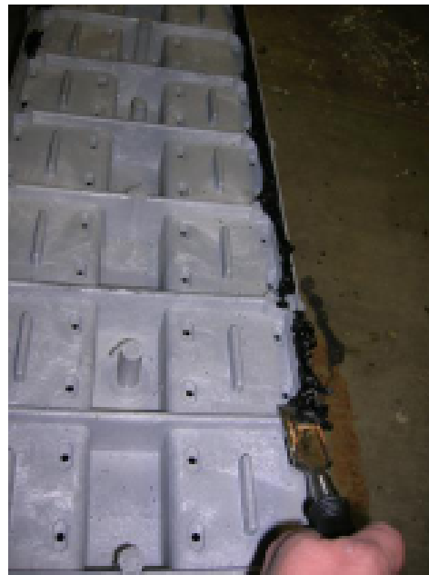
Picture #3: Removal of 3M sealant from underdrain
