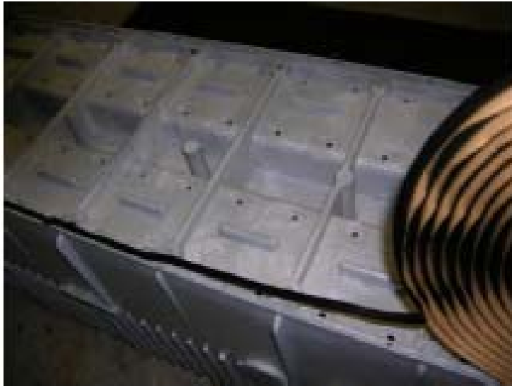
Pictures #4 & #5: New 3M sealant application to underdrain
