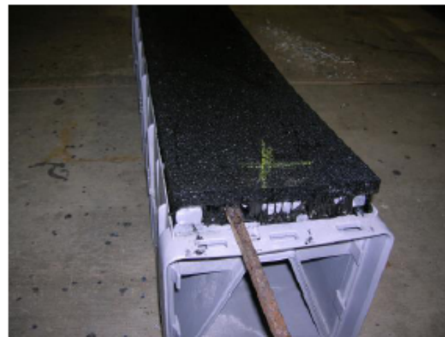
Pictures #1 & #2: Cap removal and separation from the underdrain
